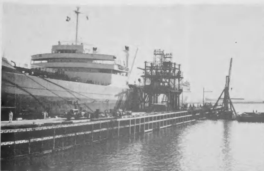
THE NORTH side of No. 1 Finger Pier underwent a major renovation recently. Timbers along the length of the pier were replaced and where mooring dolphins were located, new sleeves for securing bolts were installed and concrete was poured over a net work of reinforcing rods.
